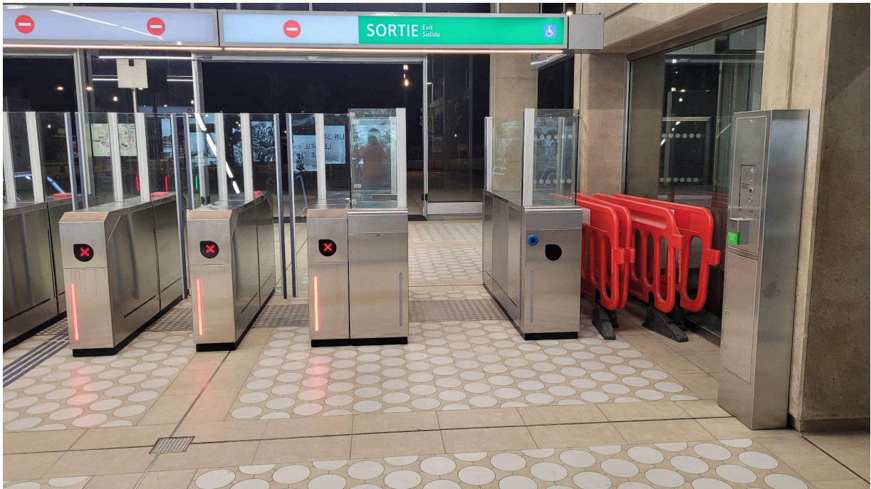
Image of a Wider Turnstile Allowing for Wheelchair Users to Pass Through
