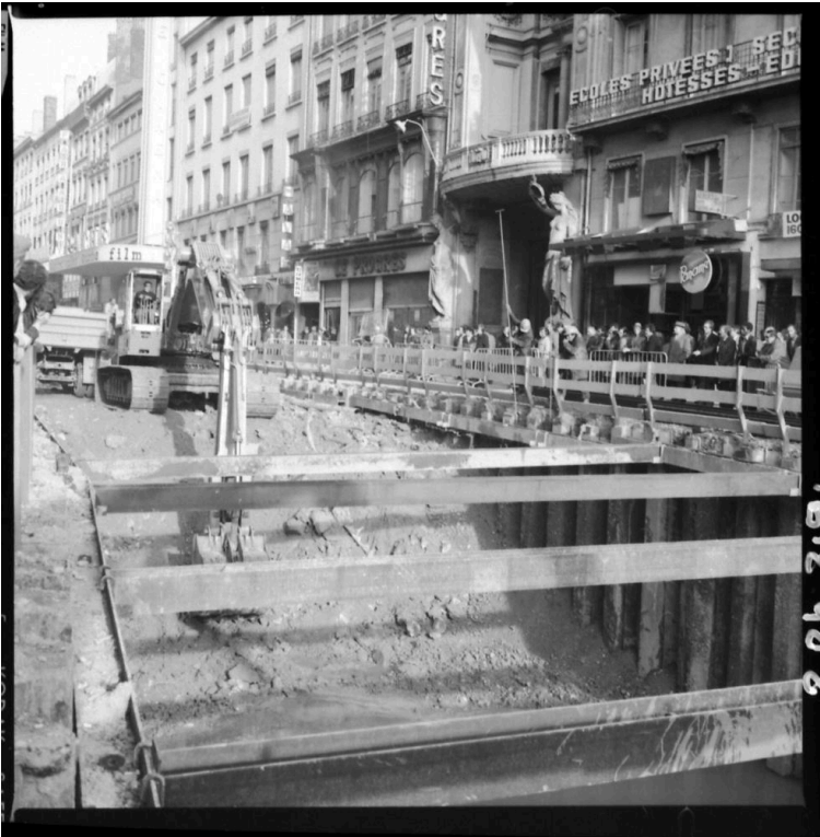
Image of the Construction of the Métro in Lyon
