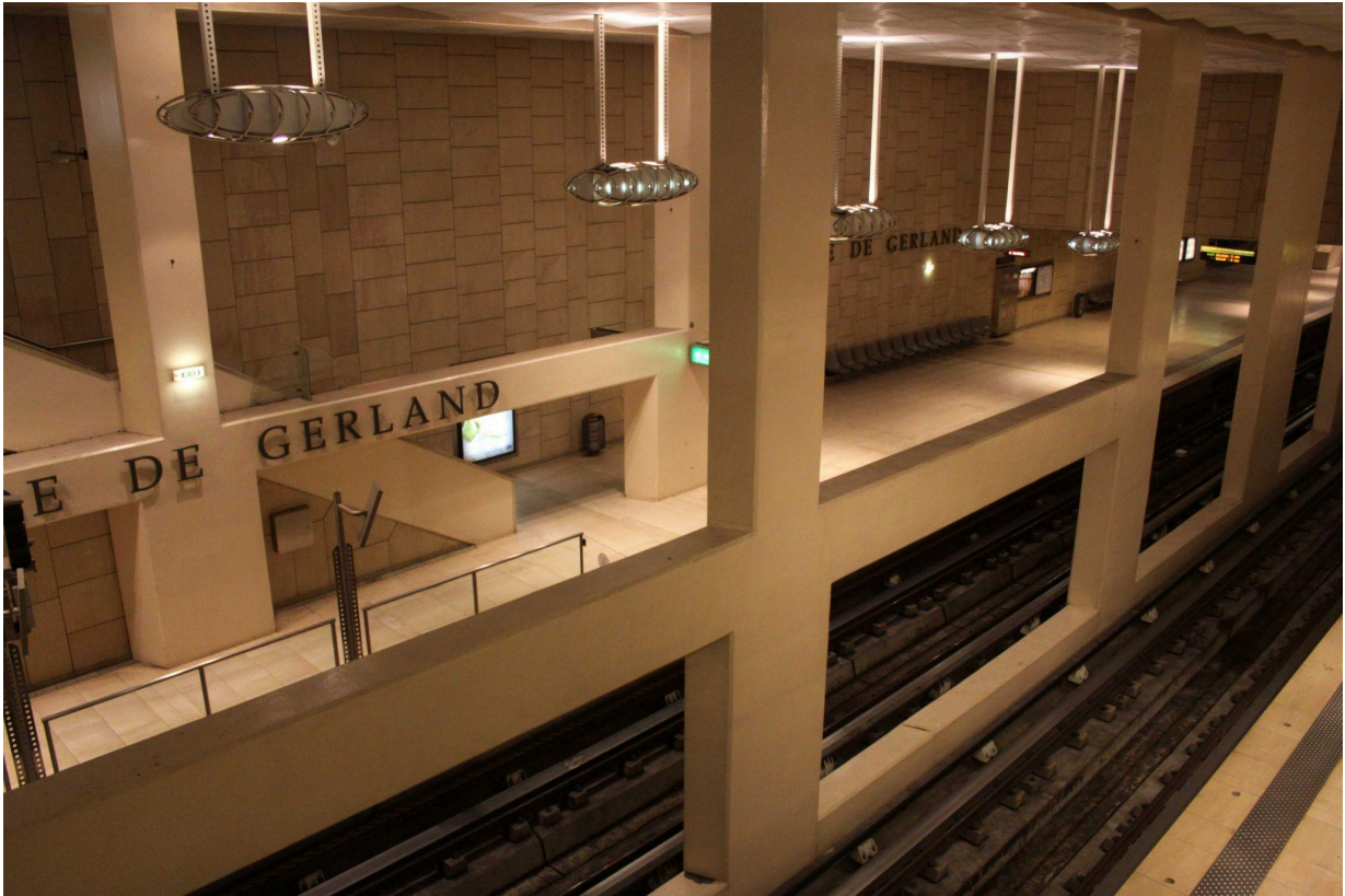
Image of a Platform in Stade de Gerland Station
